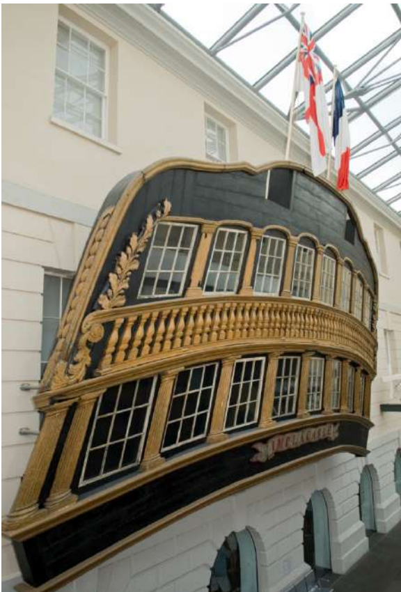
There was a much plainer style of carving after the Admiralty decided to 'explode carved works' in 1795. This is the stern of the 74-gun Implacable, captured from the French at Trafalgar and refitted in the Royal Dockyards.
