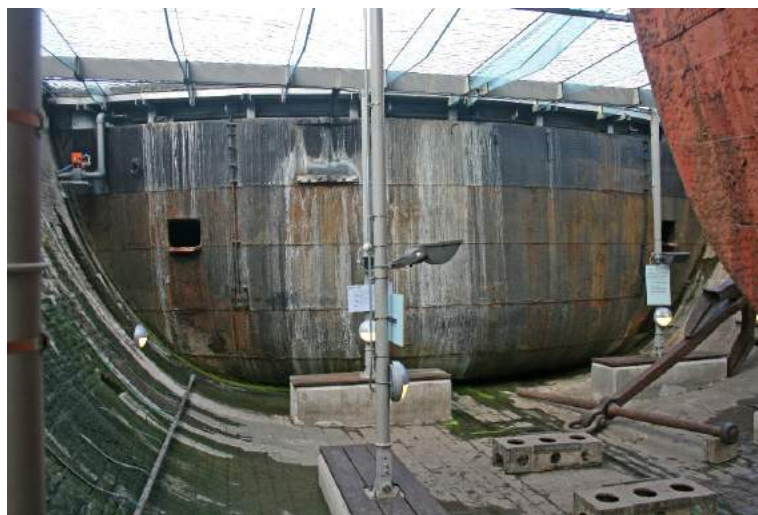
The caisson in the dock where the Great Britain is preserved in Bristol
