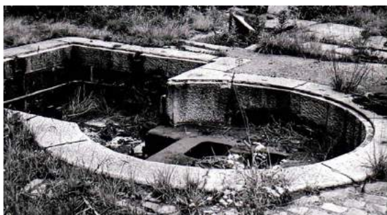
The distinctive keyhole-shaped fit of a hydraulic capstan of c 1880. Note the excellent granite masonry.
