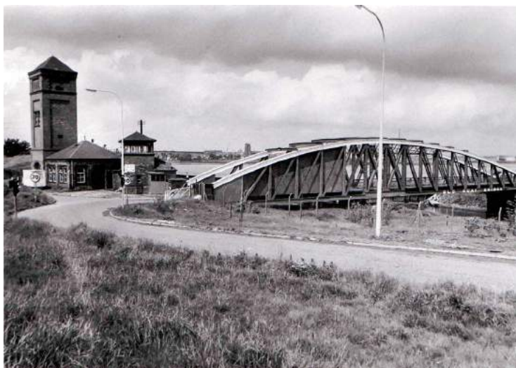
Hydraulic centre-point swing bridge across the Manchester Ship Canal. The tower on the left houses the accumulator.
