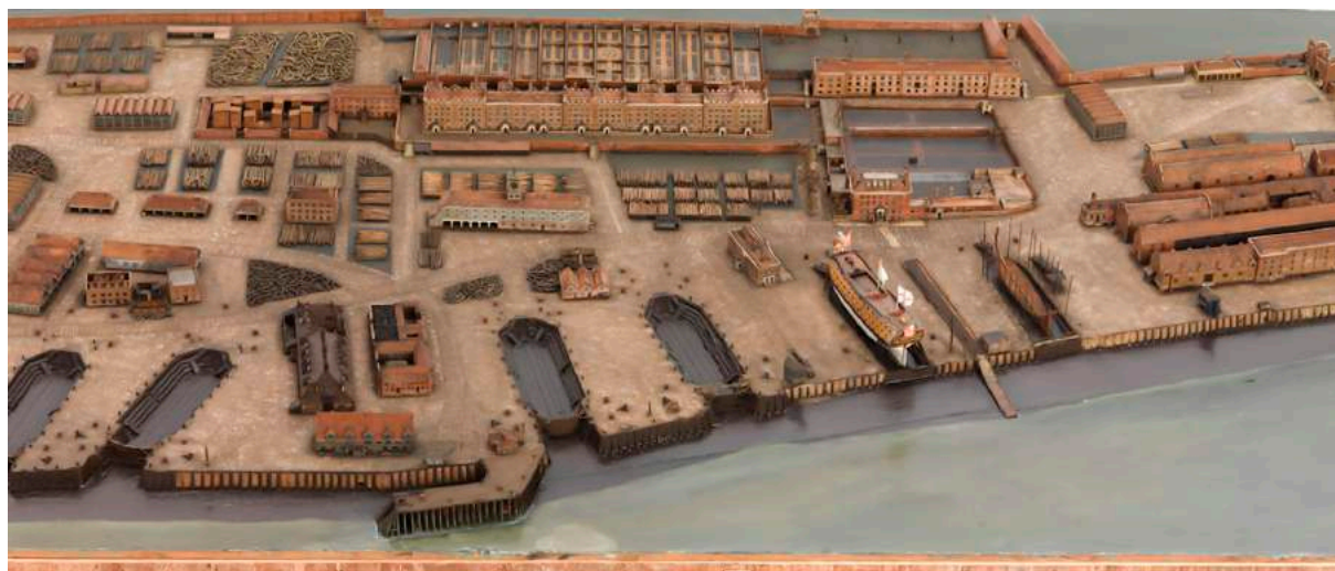
A topographical model of Chatham Dockyard c 1774, showing four empty dry docks (known as graving docks in commercial ports) to the left, with two building slips showing ships in different stages of construction.
