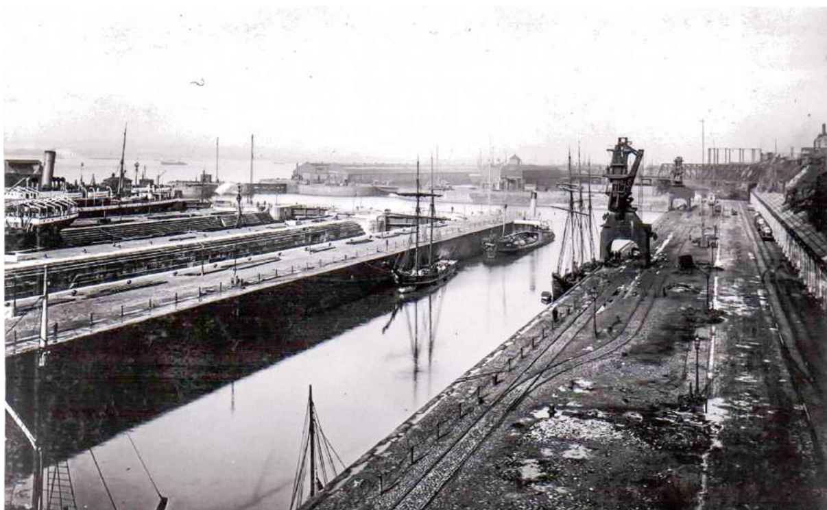
Herculaneum Dock, Liverpool. There are four graving docks to the left, while in the middle is a lifting dock with heavy lift cranes for fitting engines, propeller shafts, etc. Just visible in the left background is the pump house.
