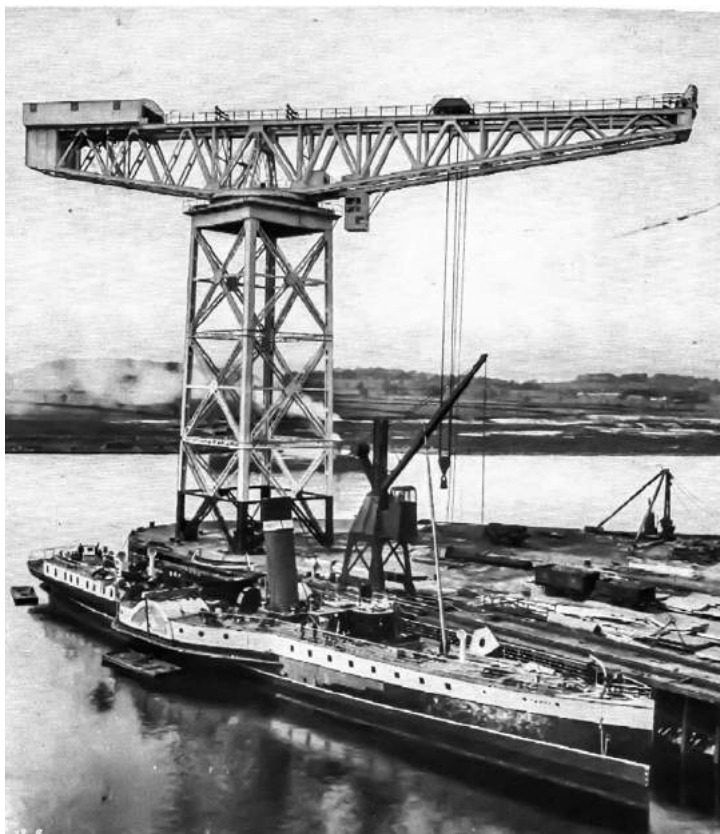
Hammerhead Crane, Cammel Laird shipyard, Glasgow from Stothert & Pitt Electric Crane Catalogue No 12 (1913) p.68
