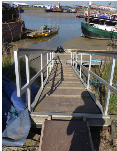
Variable gradients and stepped access on board
