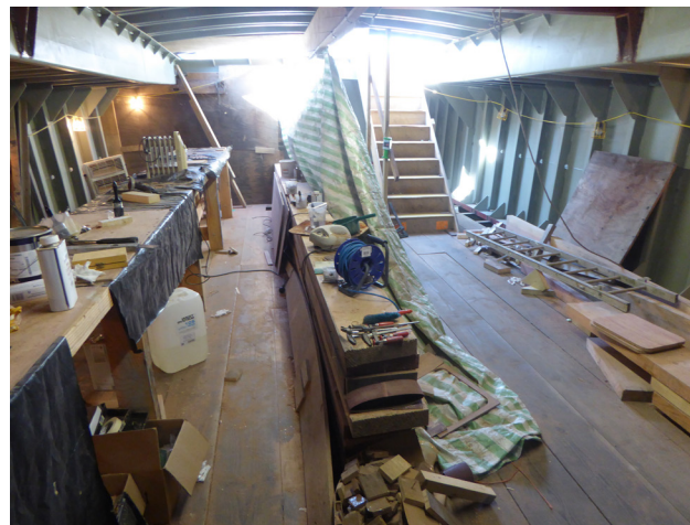
Main hold awaiting fit out
