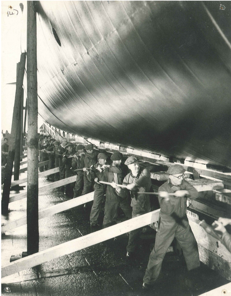
Shipwrights at Chatham 'knocking up the wedges' immediately prior to the launch of an O-Class submarine. PHA7727 © Chatham Historic Dockyard Trust
